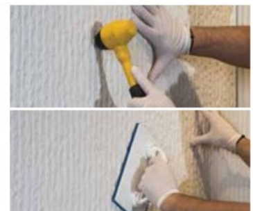
5. The panel is mounted on the wall, and the assembly process is completed with the help of a plastic hammer and sponge trowel to ensure it is firmly fixed.
