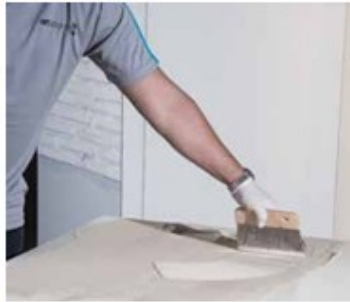
4. The prepared mixture is distributed evenly behind the panel with the help of a 3 mm metal comb.
