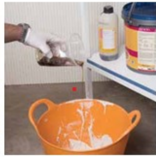
2. Mix the hardener and polyurethane adhesive thoroughly at a ratio of 10/1.
